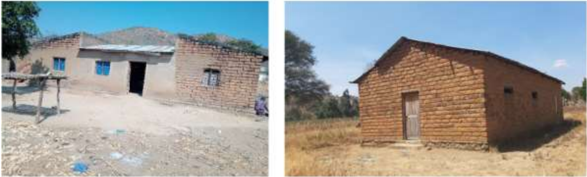
Figure 5: Some of the Houses located in the Transmission Corridor
